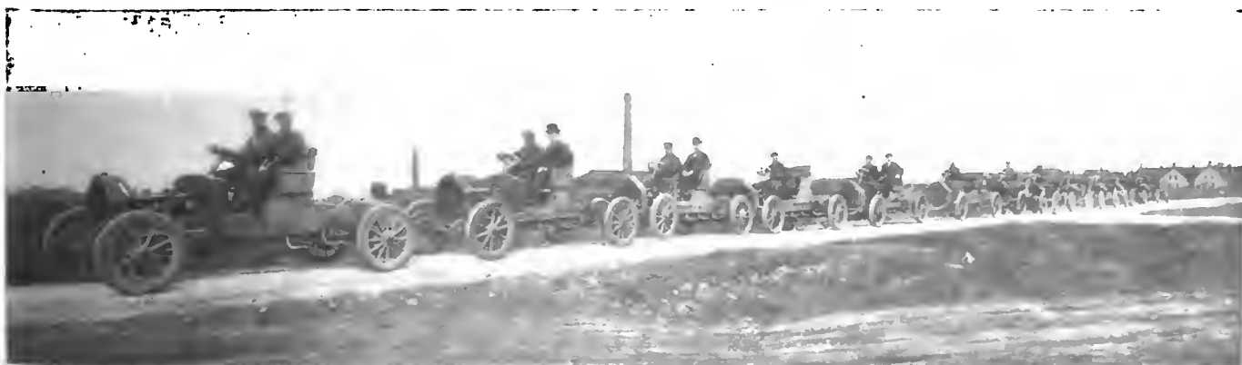
POPE-TOLEDO TESTING CREWS STARTING FROM THE FACTORY FOR THEIR DAY'S WORK.
